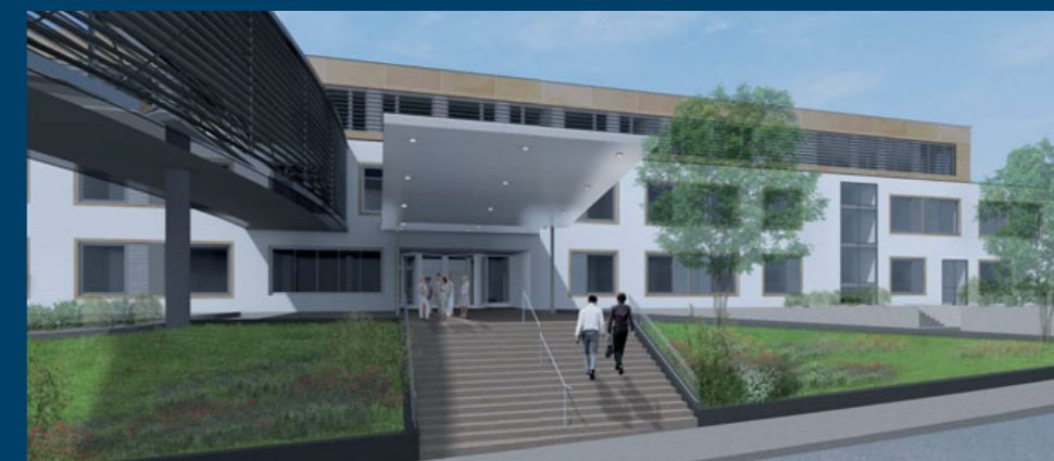
→ Landeskrankenhaus Hall in Tirol
