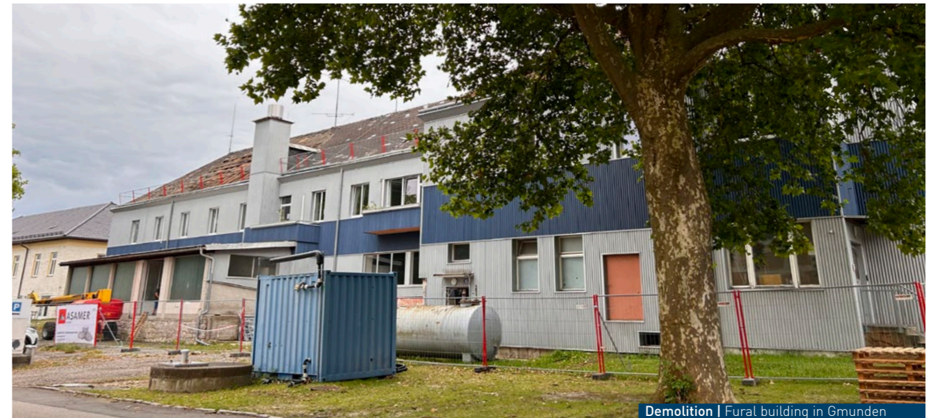
Demolition | Fural building in Gmunden
