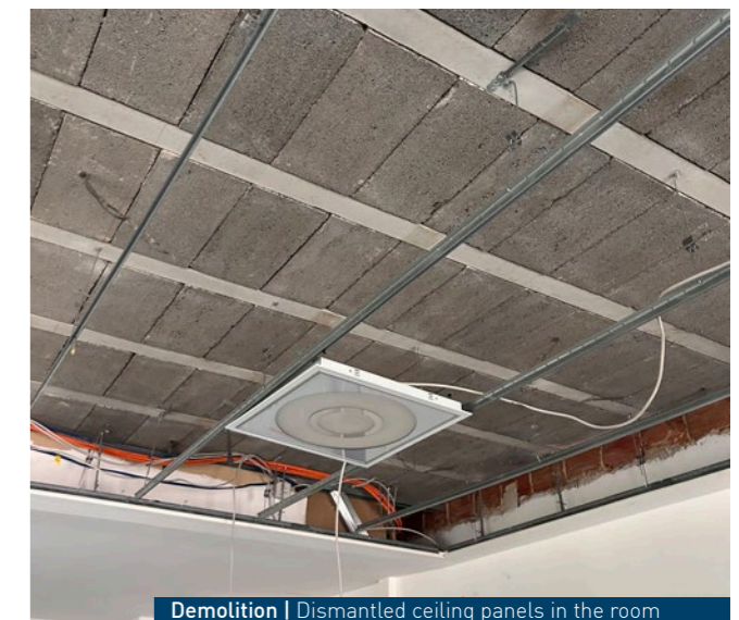
Demolition | Dismantled ceiling panels in the room
