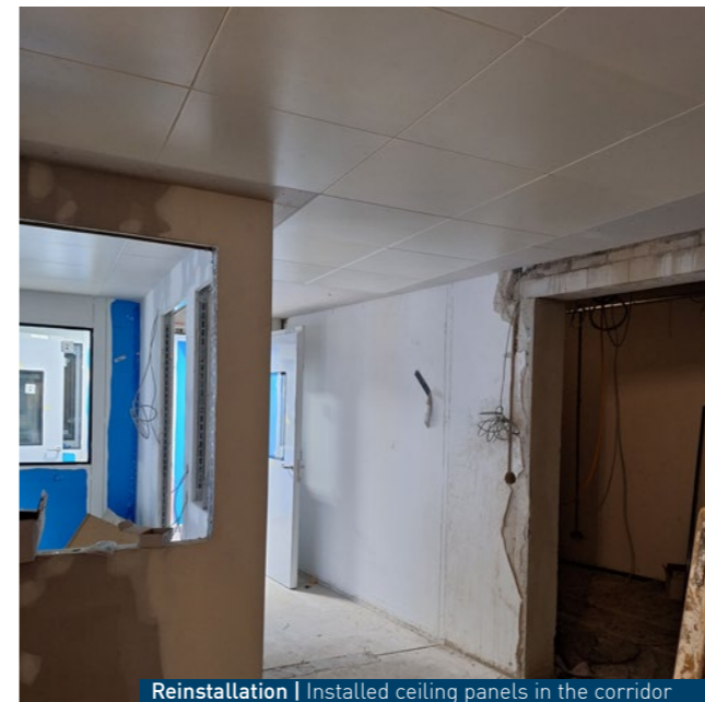
Reinstallation | Installed ceiling panels in the corridor
