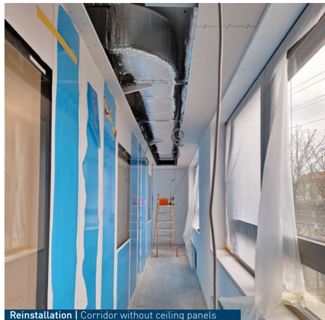
Reinstallation | Corridor without ceiling panels
