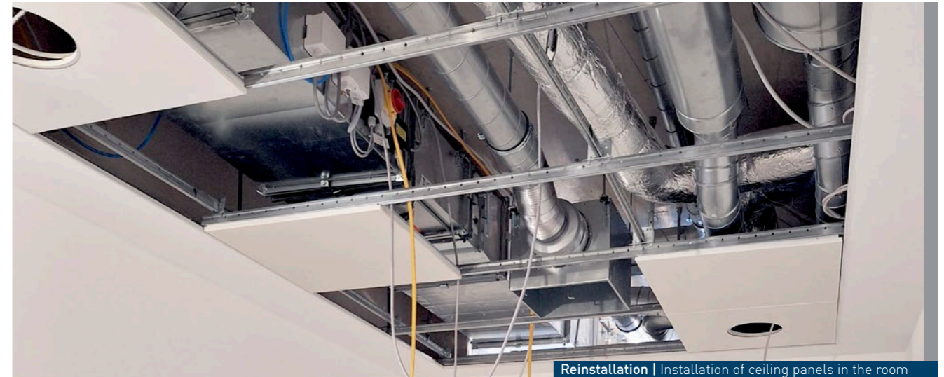
Reinstallation | Installation of ceiling panels in the room
