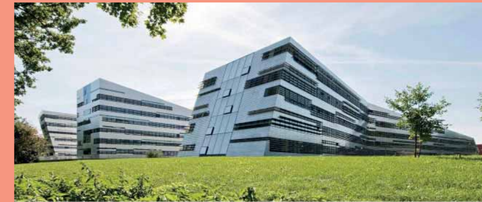
→ Education AT Johannes-Kepler-Universität Linz Controsoffitti radianti
